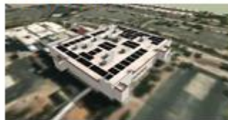
Solar Plans at Intel Chandler, Ariz.
