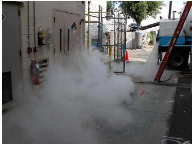
LIN Vapors Drawn Into Gas Bunker
