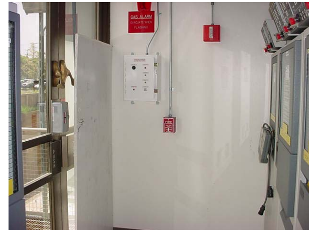
Sunlight Onto Gas Cabinets
