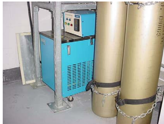
Chiller/Heater Compressor Vent
