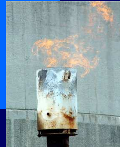
Methane flare at a WWTP
