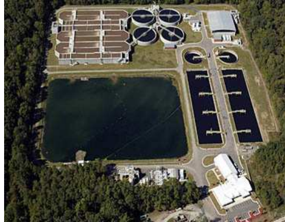
Triangle Wastewater Treatment Plant Durham, NC
