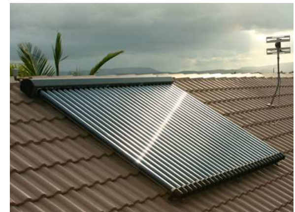
Evacuated Tube Hot Water Collector Installed by The Solar Guys, Australia
